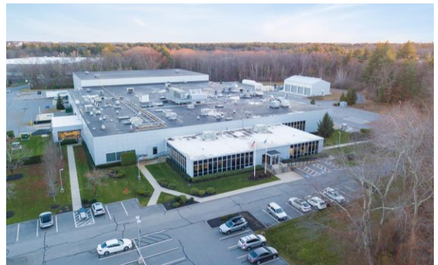
Andover Energy Exterior
